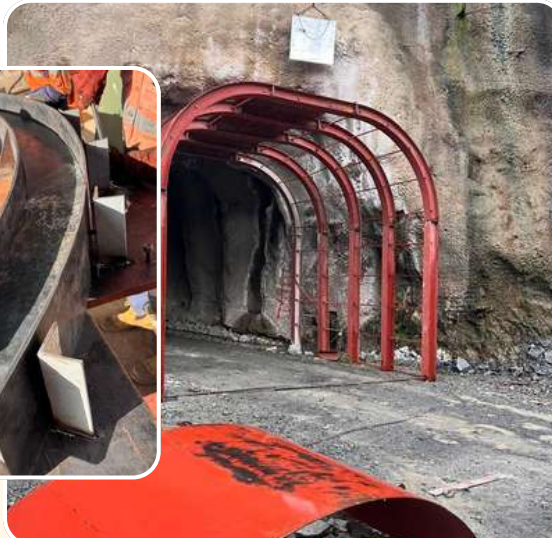
Portal Fabrication and Installation
