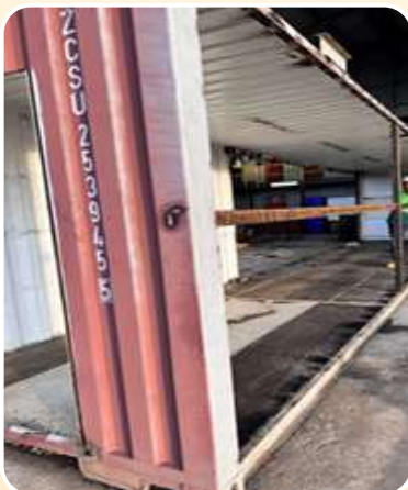
Converting Containers to Water Tanks for North Mara Underground
