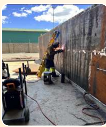
Converting Containers to Water Tanks for North Mara Underground
